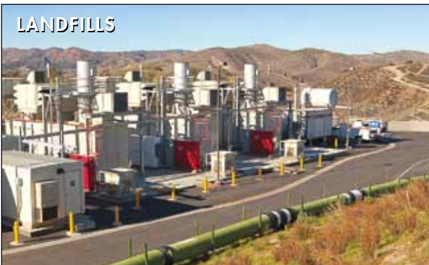
Three Mercury™ 50 generator sets running off landfill methane gas. Los Angeles County Sanitation Districts' Calabasas gas to energy facility. Agoura, California, U.S.A.
