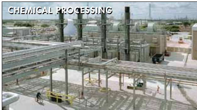
A leading industrial manufacturer in Deer Park, Texas, U.S.A., commissioned four 5.2 MW Taurus 60 generator sets to provide steam and electricity.
