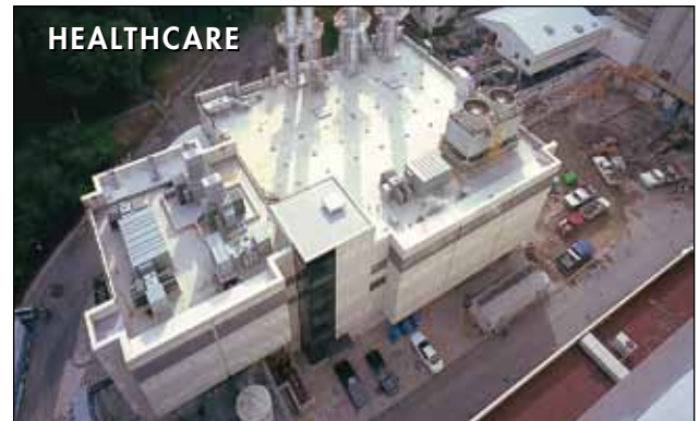
This cogeneration power plant, featuring two 5.2 MW Taurus 60 generator sets, serves a university medical center in San Francisco, California, U.S.A.
