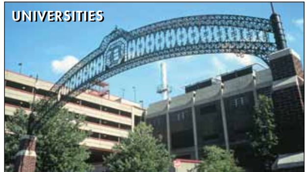
A 5.2 MW Taurus ™ 60 generator set with SoLoNOx ™ technology provides power and steam for a university campus in Pittsburgh, Pennsylvania, U.S.A.
