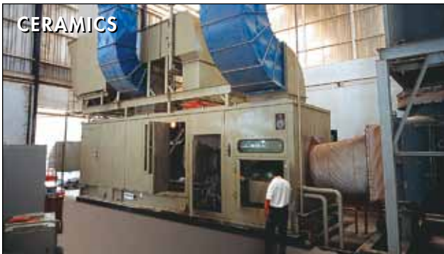
This ceramic products manufacturing plant in Surabaya, Indonesia, relies on a cogeneration system powered by a 4.6 MW Centaur® 50 generator set.
