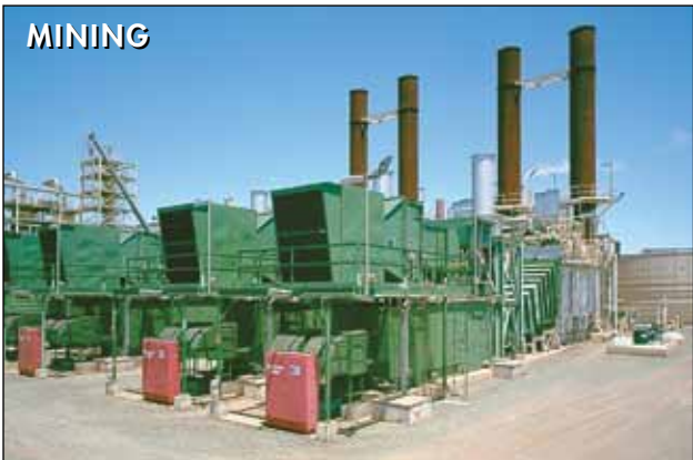
Four 5.2 MW Taurus 60 generator sets provide steam and electricity at this mine in Western Australia. Solar also provides asset management services at the facility.
