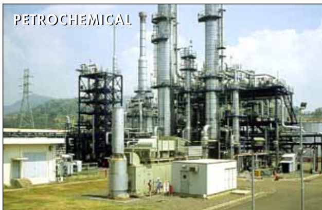
A 3.5 MW Centaur 40 generator set provides electrical power and cogeneration for this petrochemical plant in Merak, Indonesia.
